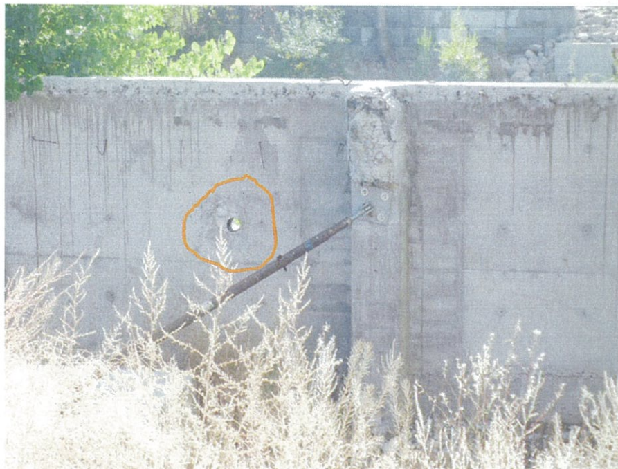
Photo taken from "inside" of demolished building.
