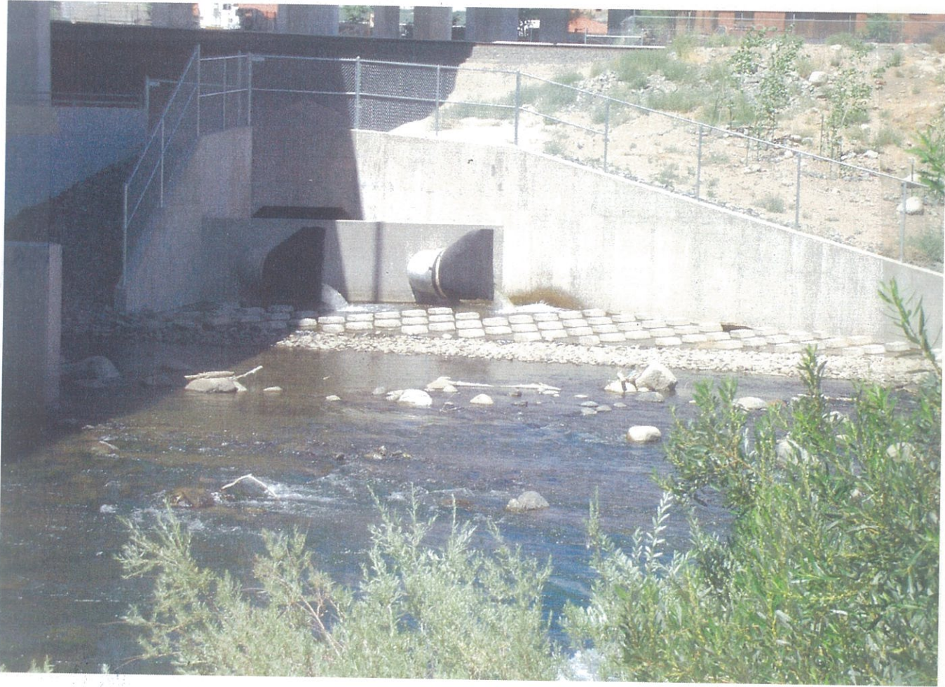
@ Wells Ave, north bank
